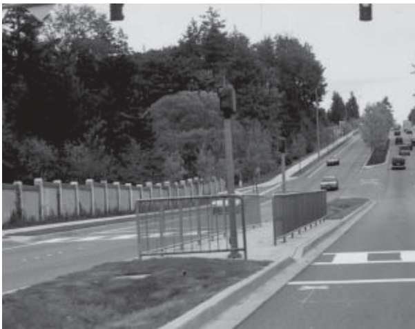
Railing is used to channelize pedestrians so they can view oncoming traffic.
