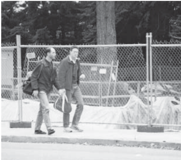
Fencing used to secure a work area supported by blocks needs to be positioned to avoid creating obstacles or tripping hazards for pedestrians.
