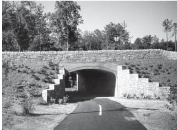
This tunnel is designed with wide openings on both ends that allows more light into the tunnel and makes it feel less imposing on pedestrians and bicyclists.
